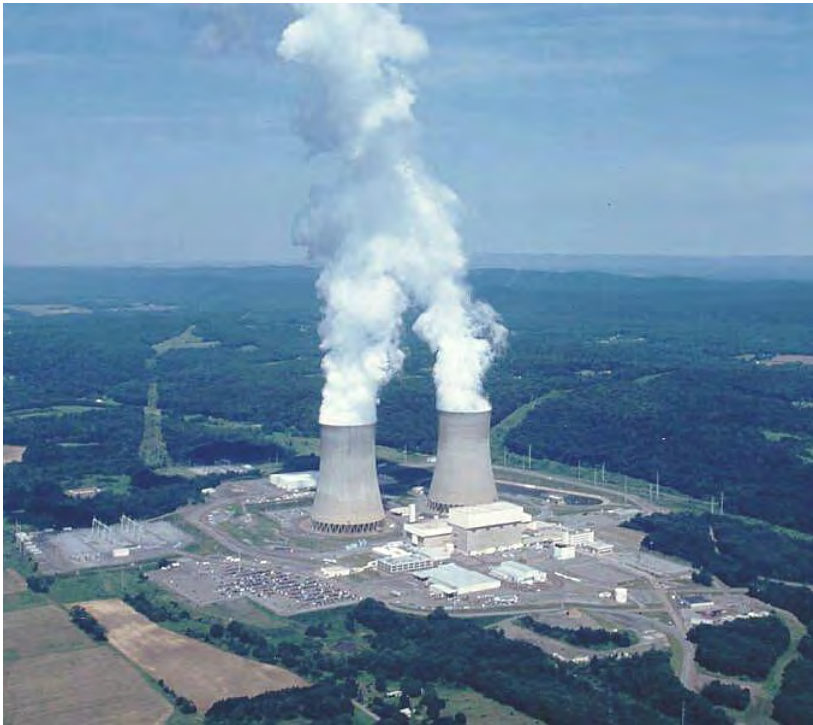
SUSQUEHANNA NUCLEAR POWER PLANT
