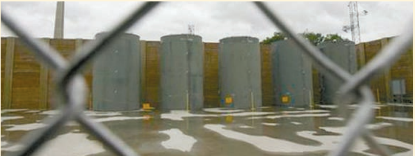
Dry-cask storage at Vermont Yankee
